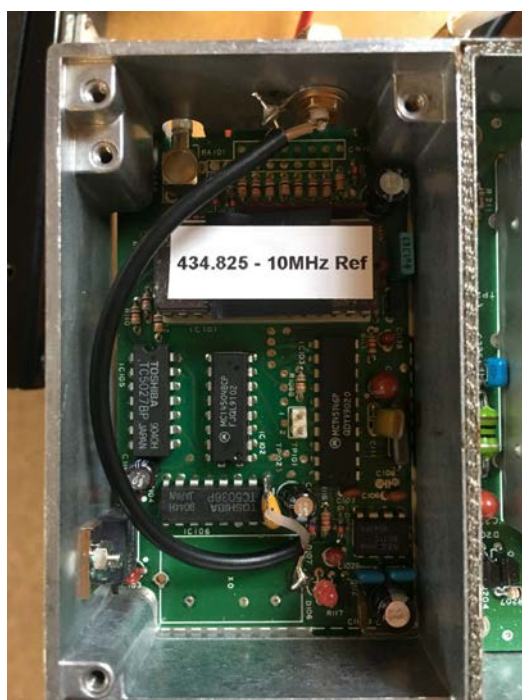
Figure 5. PLL compartment of the KL receiver
